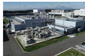
The completed Kiyohara Smart Energy Center (Utsunomiya City, Tochigi Prefecture)
