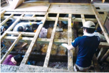
Recovery volunteer activities in an area damaged by flooding during the typhoon
