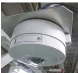
A monitoring camera
